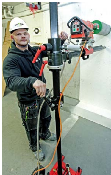
Horizontal drilling using 50 + telescopic drill stand and Weka core drill motor.
